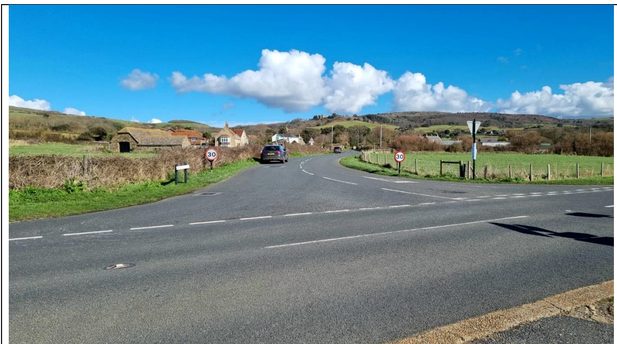
Military Road has a major / minor junction with Brook Village Road which has a significantly flared approach
